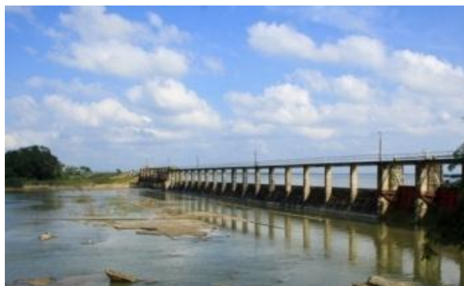
Fig 1.2 Iranamadu Irrigation Scheme
